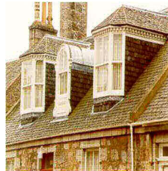
Above: Examples of the variety of dormer types to be seen around Aberdeen
