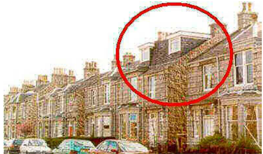
Above: Example of a poorly designed roof extension – Dormers are too large, dominating the roof slope, and use of substantial infill panels and slated aprons contributes to bulky appearance
